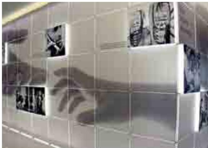
Lounge area wall in constructiv pila petite: Another area features constructiv pila petite which serves as a dividing wall between the office and visitors' lounge. constructiv pila petite spans a distance of more than 10 m with a height of 3.5 m without trussing. The wall is secured to a hanging steel beam and tensioned to the concrete floor below. The rigidity of the wall is further strengthened by integrated wall panels decorated with bold texts and lifestyle images.
